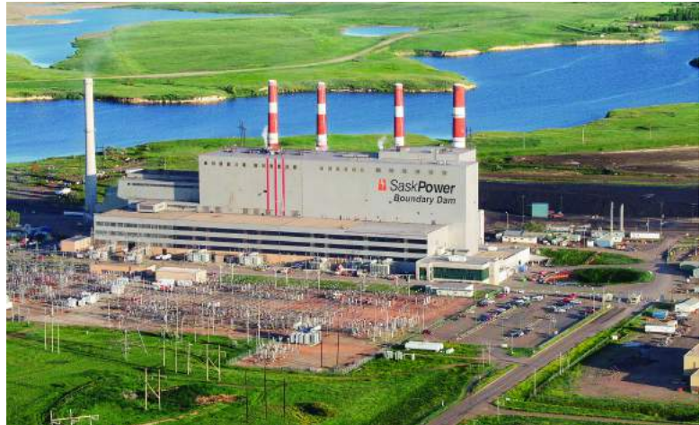
Sask Power's Boundary Dam power plant in Canada was the world's first commercial scale CCS plant. Image: Sask Power, creative commons license
